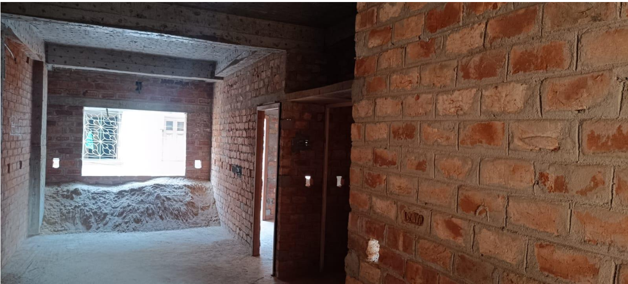
Internal Construction/Infrastructure Photo
